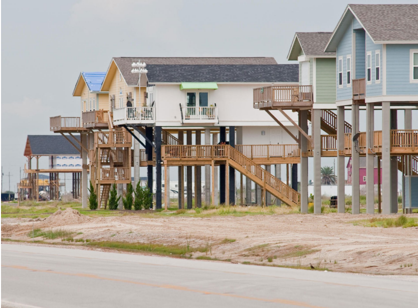
Homes that survived the ~20-foot-high storm surge of Hurricane Ike in Bolivar Peninsula, near the community of Caplen. Image: TWDB
